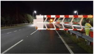
An automatic taper which can close off lanes in minutes and saves road workers having to put out cones in the face of oncoming traffic is to be trialled on the National Highways network.
