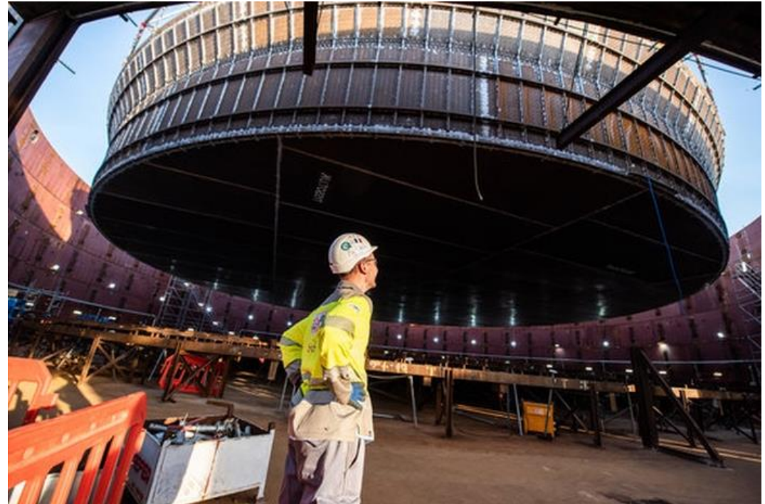
The world's largest crane, dubbed 'Big Carl' has lifted a 170t steel containment liner used in the construction of the second reactor at Hinkley Point C nuclear power station into place.
