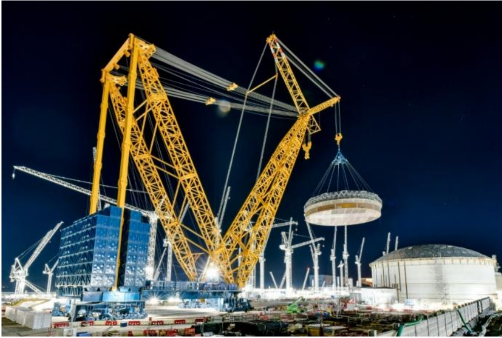
The world's largest crane, dubbed 'Big Carl' has lifted a 170t steel containment liner used in the construction of the second reactor at Hinkley Point C nuclear power station into place.
