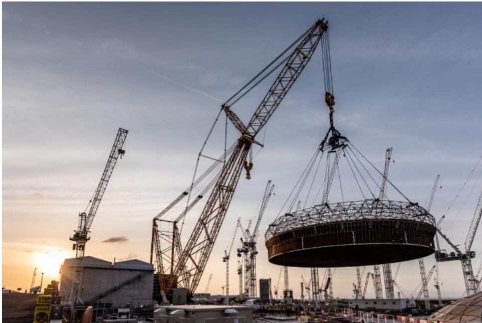
The world's largest crane, dubbed 'Big Carl' has lifted a 170t steel containment liner used in the construction of the second reactor at Hinkley Point C nuclear power station into place.
