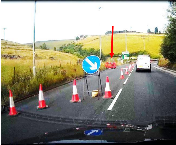
Coned area with excavation arrowed
